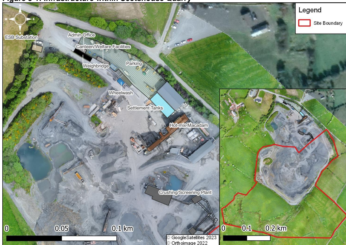
Figure 3-1: Infrastructure within Scotshouse Quarry
