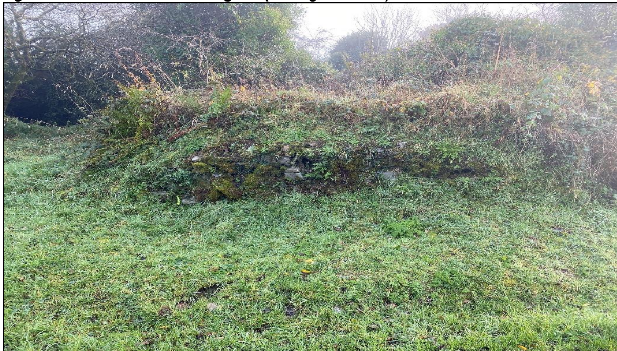
Figure 13-10: Remnants of Building Ten (looking southeast)
