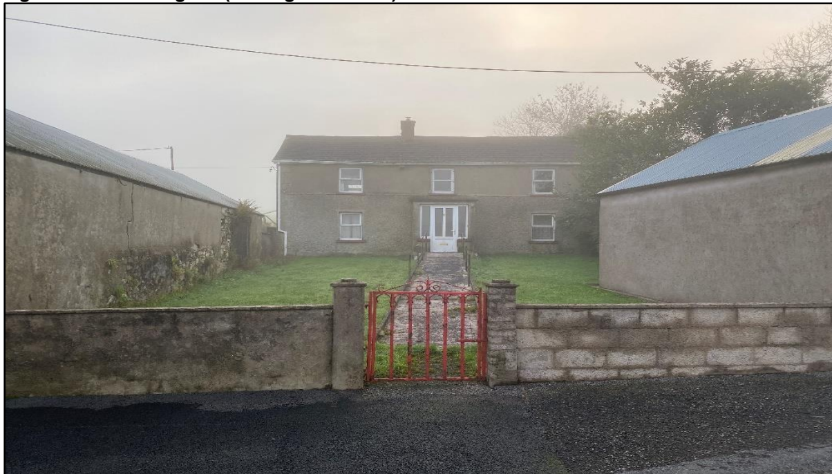
Figure 13-4: Building Six (looking southwest)
