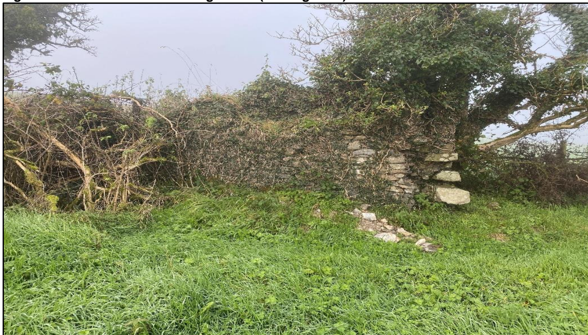
Figure 13-5: Remnants of Building Seven (looking west)
