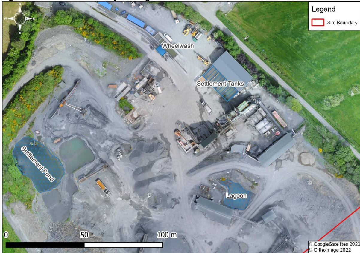
Figure 3-8: Scotshouse Quarry Drainage
